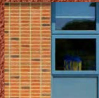
Gebrik's insulating properties will help to significantly improve a building's thermal performance (it is proven to reduce a building's U-value by up to 60%) and keep wall thickness to a minimum. The insulating material is polyurethane (PUR) and uses pentane as its blowing agent and therefore does not release CFC or HCFC agents during manufacture. The PUR has a BREEAM element number of 815320017 and Green Guide rating of A.
