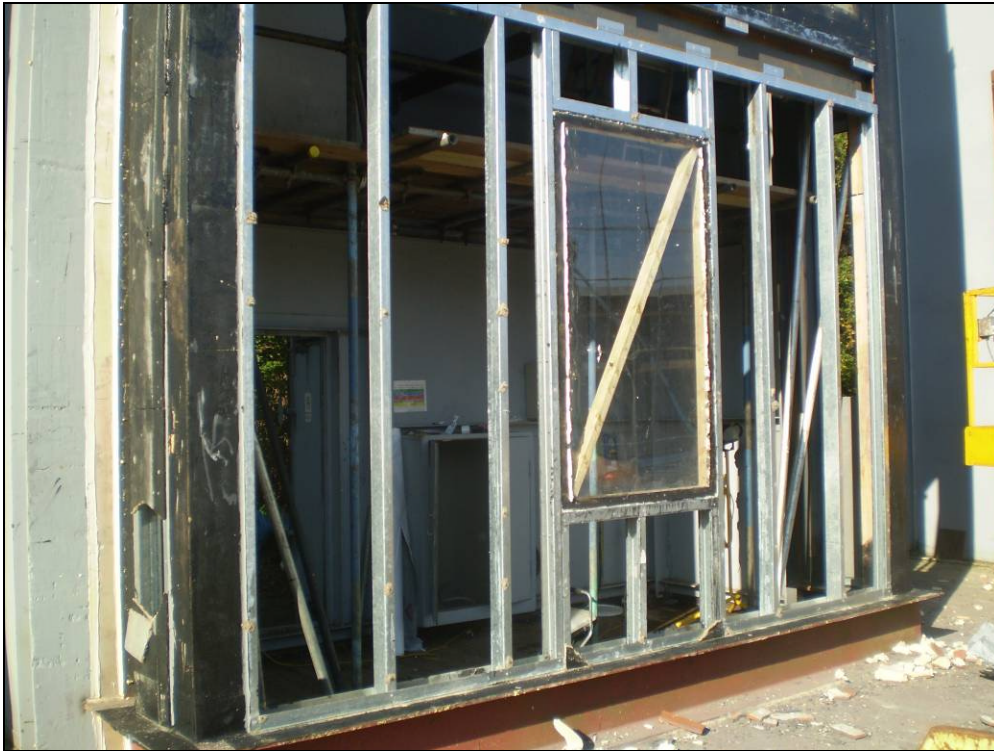
METSEC FRAME AT LOWER LEVEL OF SAMPLE
