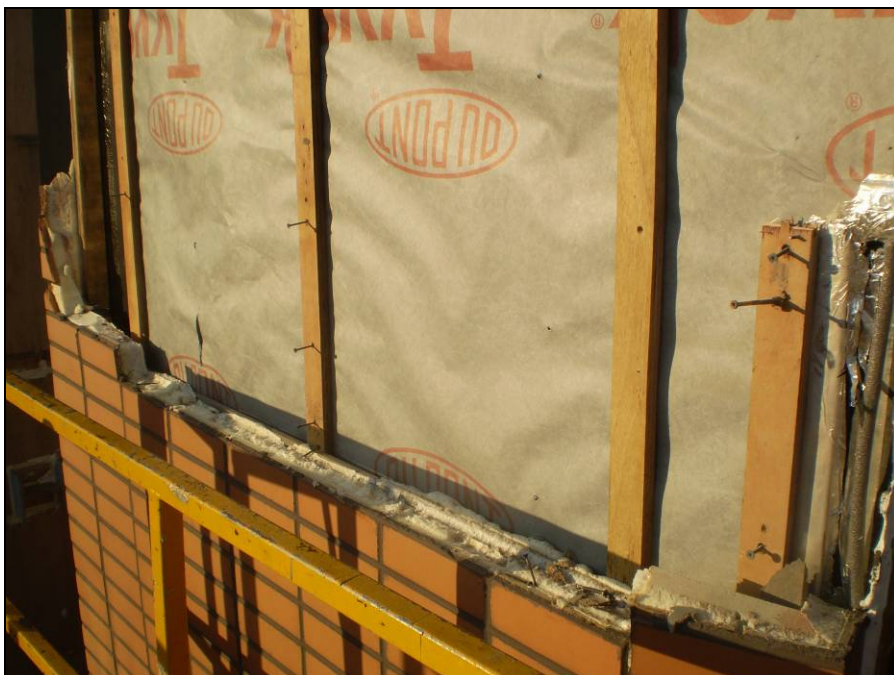
UPPER GEBRIK PANELS REMOVED
