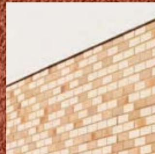
The composite panels and corners comprise of 15-20mm thick frost-resistant, clay brick slips, cast in polyurethane insulation and are supplied in Stretcher, Stack, Flemish or other bond formats. There is a range of approx 700 different brick choices in a variety of finishes and sizes; samples and details of which are available upon request. Alternatively, non-standard brick finishes can be developed subject to quantity and agreement with the manufacturer.
