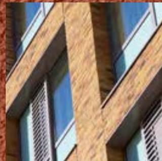
Designed to create a lightweight, natural brick appearance, Gebrik insulates and protects a building from water penetration and is site-applied to buildings constructed of masonry, timber, steel frame or SIPs to clad new buildings or refurbish existing buildings.
