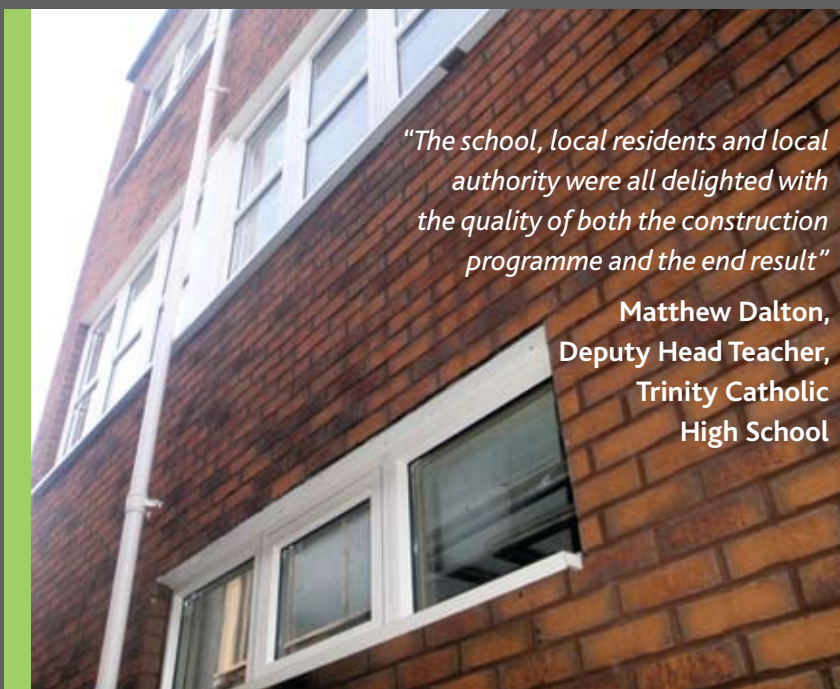
Extruded brick returns were applied on site to create a true brick facade
