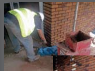
Gebrik being pointed using a mechanical pointing system
