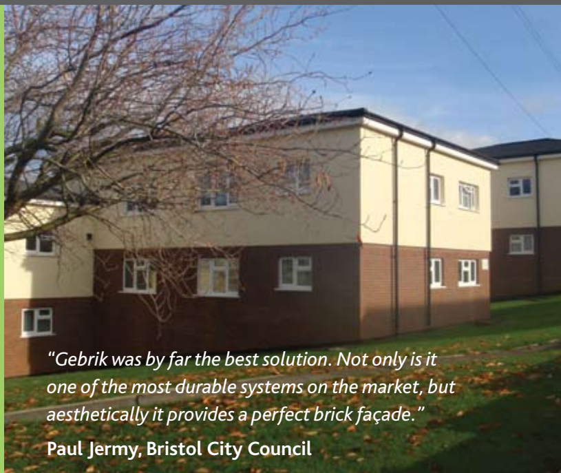
Brick slips 'stitch' the panels together to maintain stretcher bond
