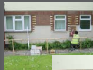
Gebrik panels are mechanically fixed directly to the existing masonry structure
